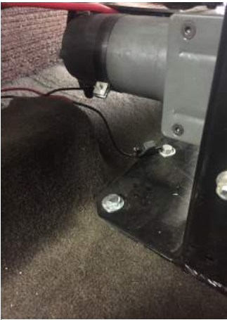
Figure 17: View Through Rear Passenger Door
